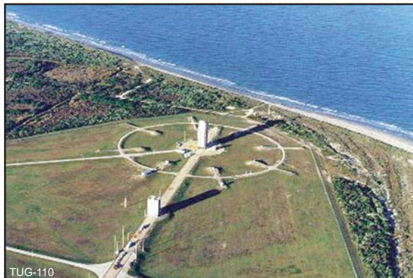
Figure 8-11. LC-46 Launch Complex.
